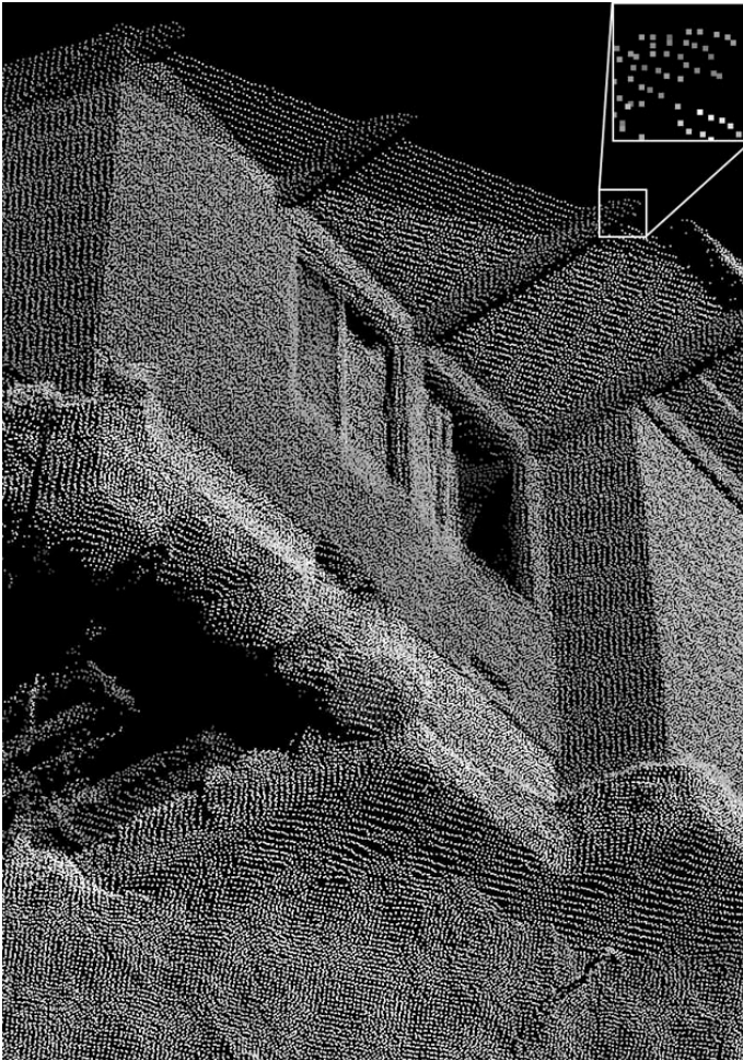
Figure 1: A T-LiDAR scan looking up through the floorboards of a house after a landslide removed part of its foundation. The inset shows a close-up of the placard-based visualization, revealing gaps between reflections.
